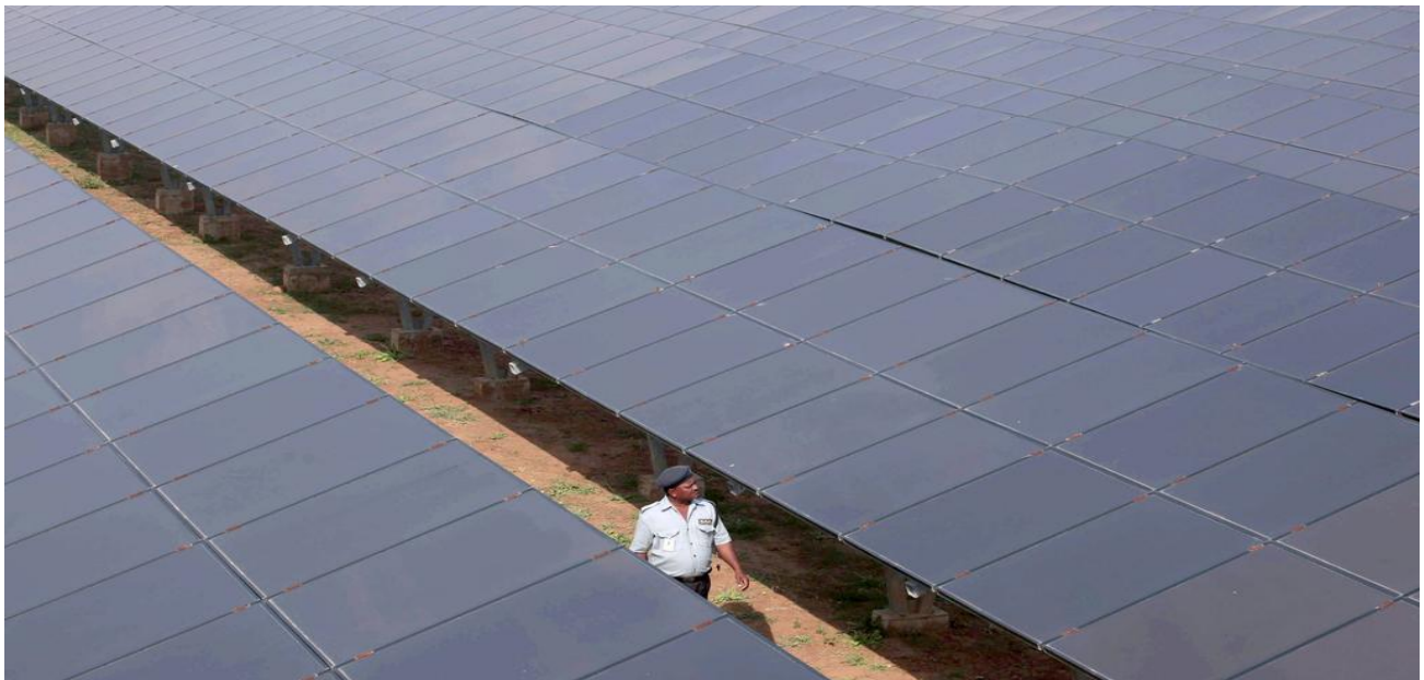
An Indian security man walks amid solar panels at a solar power project site in Raisan village near Gandhinagar, India. Ajit Solanki / AP Photo
